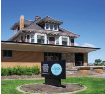
Example of business space added to single family residential on W. 14th Street: "All Things for You". This typology can be typically found within the neighborhood.
