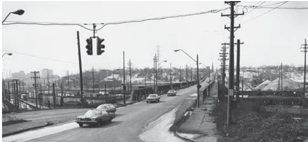
Clark Avenue bridge crossing over the railroad tracks between Quigley and W. 3rd Street. Tremont History Project.
